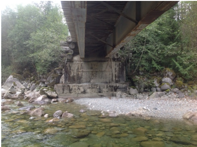
Left Bank Abutment when facing downstream
