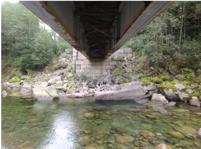
Right Bank Abutment when facing downstream
